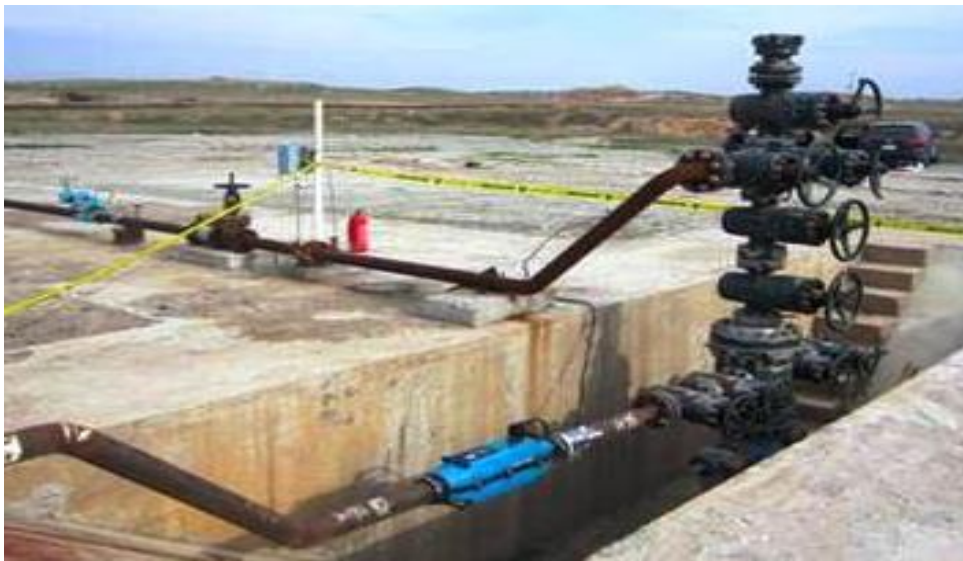
PassiveSONAR™ meter on production pipework (foreground) and ActiveSONAR™ meter on injection side (background)
